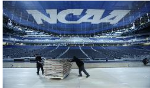
Workers at Detroit's Ford Field on Thursday move a pallet of basketball court flooring that will be installed for this weekend's Final Four games.
